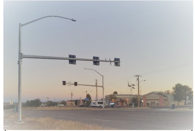
Photo Credit: Dennis Donovan, P.E. SVMPO Civil Engineer
