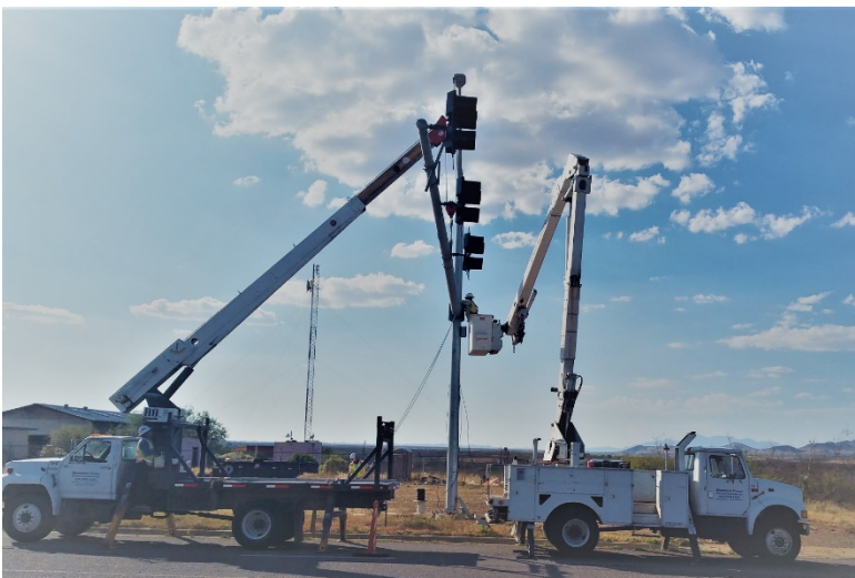
Photo Credit: Dennis Donovan, P.E. SVMPO Civil Engineer
